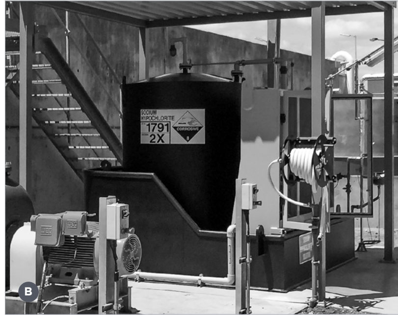
C Right-side shot: Another perspective of the custom panel, tank & bund. The chemical storage tank contains sodium hypochlorite which is used for dosing water in WA's southwest region.
