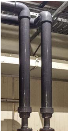
UPVC Pipework installation at the Dairy Plant
