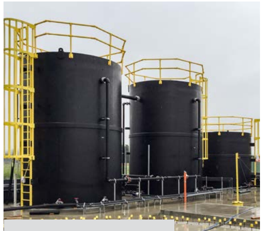
The tank installation complete.
