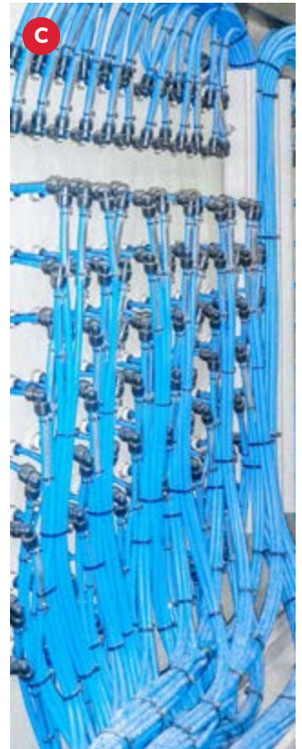
C The reverse side of the panel showing organised tubing.
