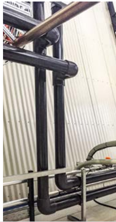
UPVC Pipework installation at the Dairy Plant
