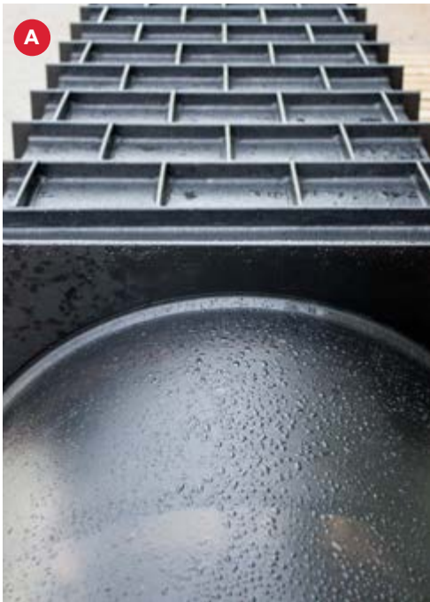
A left: large bore PE end in the foreground shows transition to the rectangular extrusion welded, reinforced, central section.
