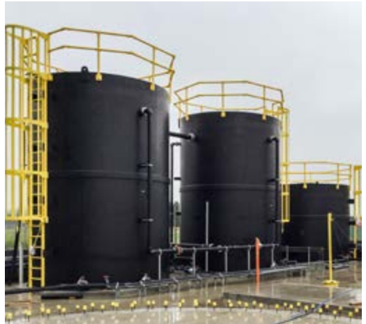
The tank installation complete.
