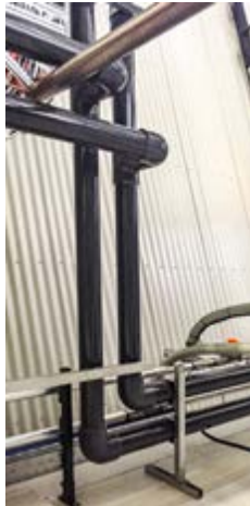
UPVC Pipework installation at the Dairy Plant
